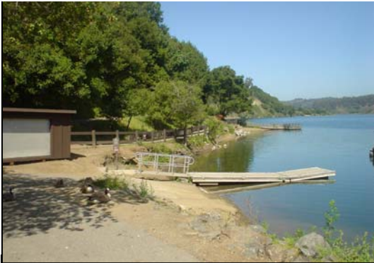
Marina trail access, floating dock & observation deck looking north
